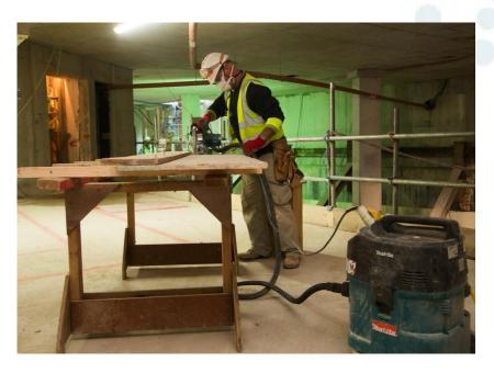
Where power tools are used on-site for wood working, dust exposure can be controlled by using local exhaust ventilation (LEV). Most commonly in construction this will involve on-tool dust extraction consisting of:
