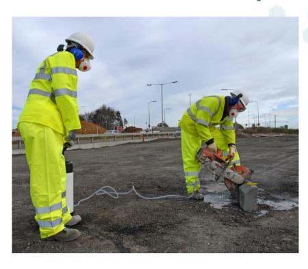
Water suppression systems fitted to tools usually involve spraying water directly onto the material. The water spray is supplied via mains water supply or a pressurised water bottle. There needs to be an adequate supply of water so make sure you have this before you start. Pouring from a container before you start will not be sufficient.
