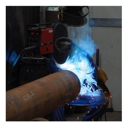
Where flexible arm fume extraction is used, the position of the extraction hood is crucial! If too far away, it has no benefit; it typically needs to be placed within 30cm of the welding source although this range may be much shorter. It is important that the system's capture range is identified during commissioning and further routine testing of the LEV system.
